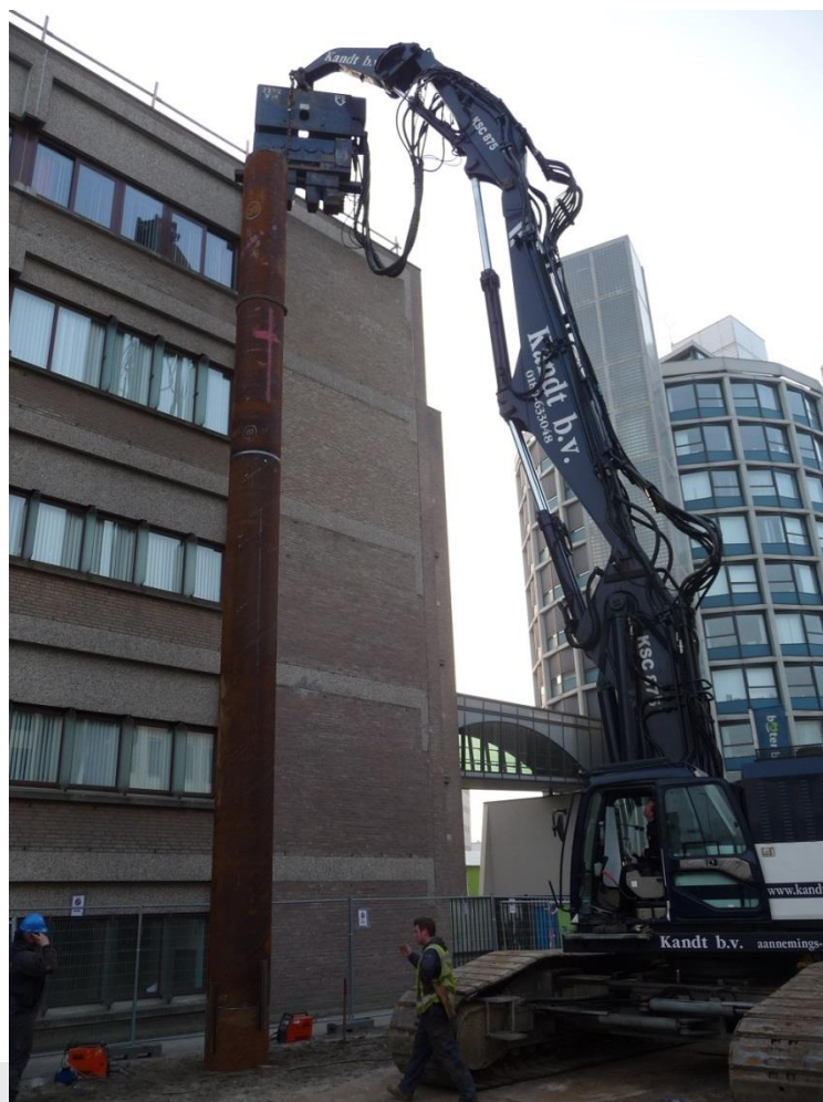
Intrillen stalen casing.
